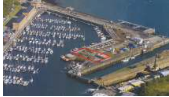
Build site at Milford (outlined in red).
